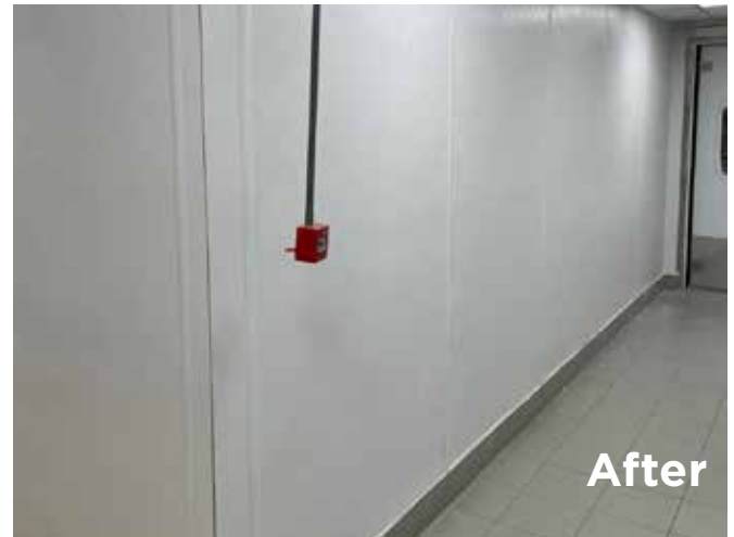
Step 4: Install Cover Profile
